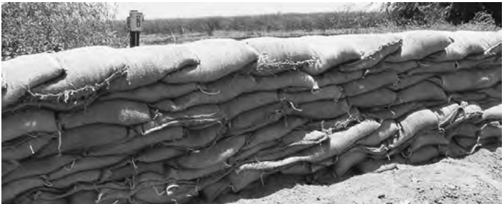
Sandbag Wall Construction
